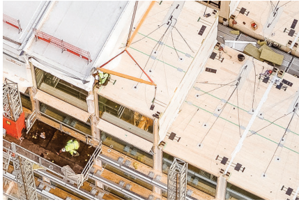
▲ Figure 2.6.13. Detail image of the installation of the individual hotel modules, showing how each module sits on the module below. © Martinsons | Jonas Westling
