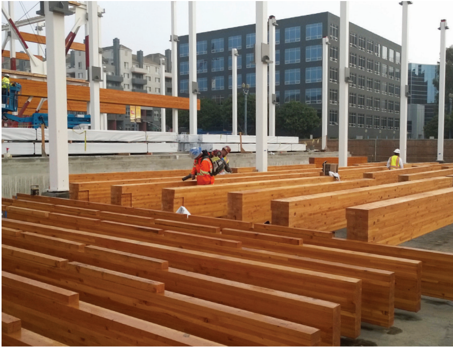
▲ Figure 2.3.11: With columns in place, the prefabricated glulam beams were brought to the site and hoisted individually. © SOM
