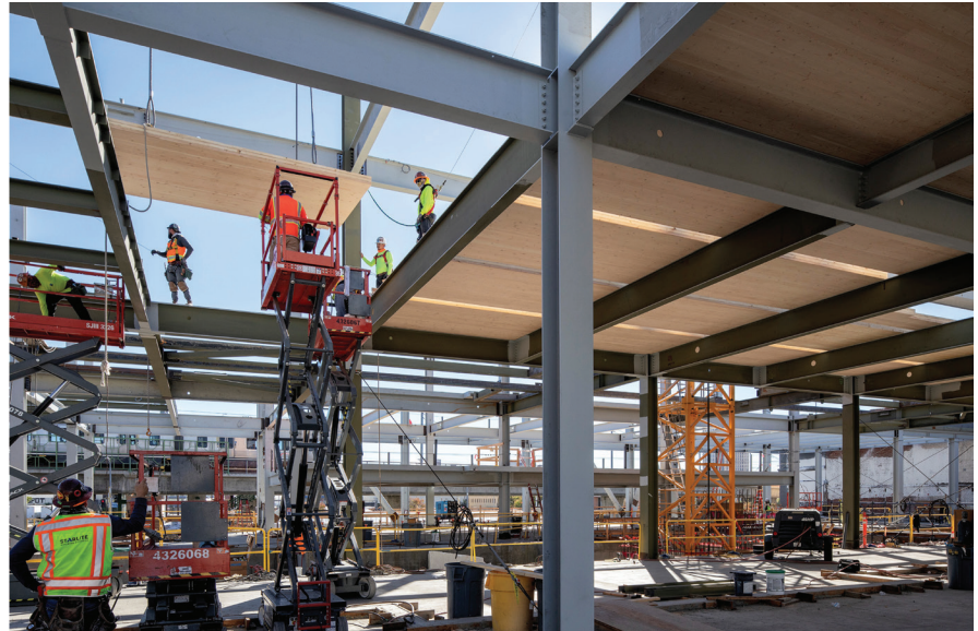
▲ Figure 2.2.8: Constructors guide a CLT floor panel towards the frame, where it will be bolted in place. © LEVER Architecture
