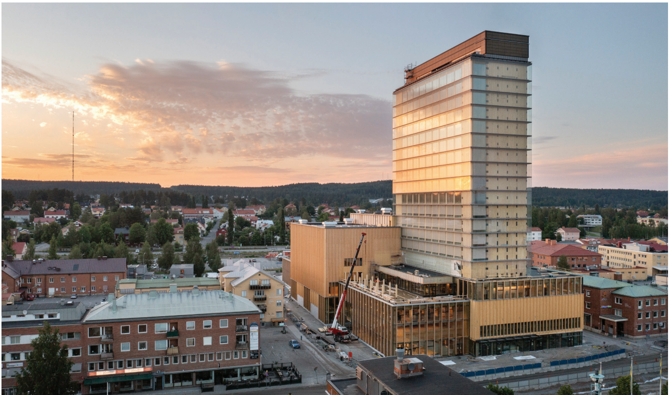
▲ Figure 2.6.23. The nearly finished project shows the impact of the double-skin façade, as installed. The final construction was a canopy on the exterior deck. © Patrick Degerman
