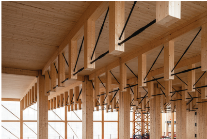
▲ Figure 2.6.7. Detail of the steel-timber truss used for the long spans of the cultural space. © Martinsons | Jonas Westling
