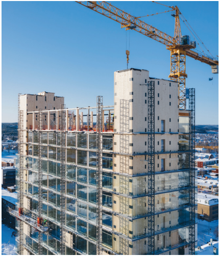
▲ Figure 2.6.12. The top two floors house a restaurant and hotel amenities, and as such required a column-and-beam structural system. © Martinsons | Jonas Westling
