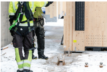
▲ Figure 2.6.9. Detail of the connection between the knife plate embedded in the concrete floor at level 1 and the GLT column. © Martinsons | Jonas Westling
