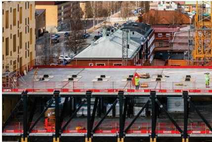
▲ Figure 2.6.14. The top of the steel truss at level 6, with knife plates integrated for easy connection to the GLT columns above. © Martinsons | Jonas Westling
