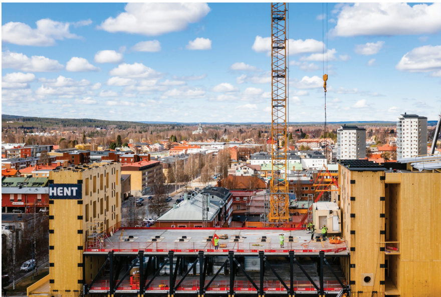
▲ Figure 2.6.21. Modules arrived on-site wrapped in plastic, which was removed once they were set into place. © Martinsons | Jonas Westling
