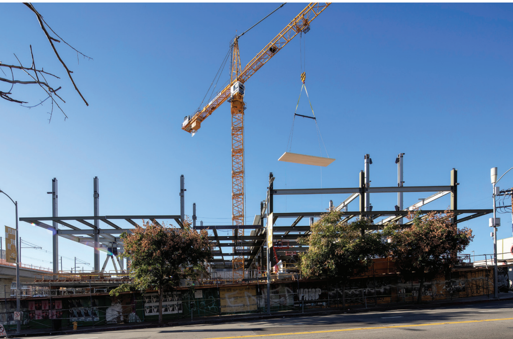
▲ Figure 2.2.7: Tower crane at site center places a CLT panel on the steel frame. © LEVER Architecture
