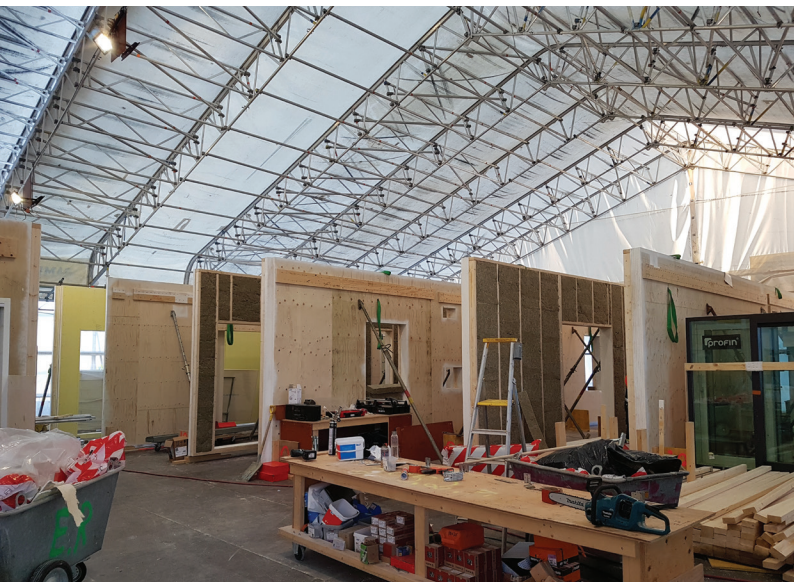
▲ Figure 2.5.8. “On-site prefabrication” of LVL wall panels involved fitting with door and window hardware in a tent. © Mika Keskisalo
