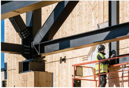
▲ Figure 2.6.6. Detail of the connection between the steel box truss and the GLT column below. © Martinsons | Jonas Westling
