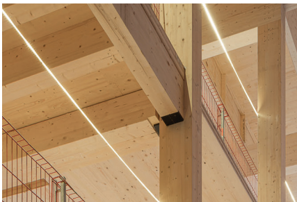
▲ Figure 2.6.8. Detail of the column-beam-platform system used on the lower floors. © Martinsons | Jonas Westling
