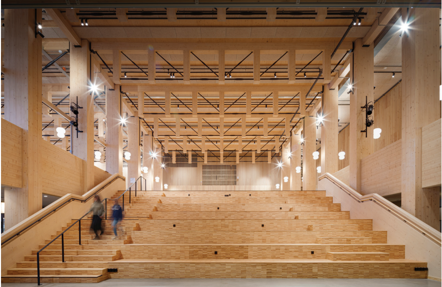
▲ Figure 2.6.11. GLT chorded trusses, augmented by steel tension rods, allow long spans over an amphitheater-style seating area on Level 1. © Martinsons | Jonas Westling
